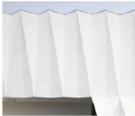
Cast pleats in concrete façade.
