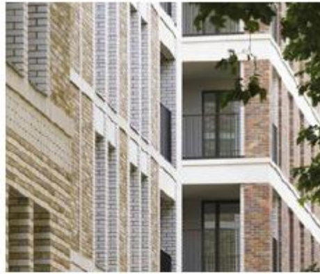
Horizontal concrete banding within brick façade.
