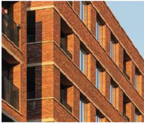
Horizontal concrete banding within brick façade.
